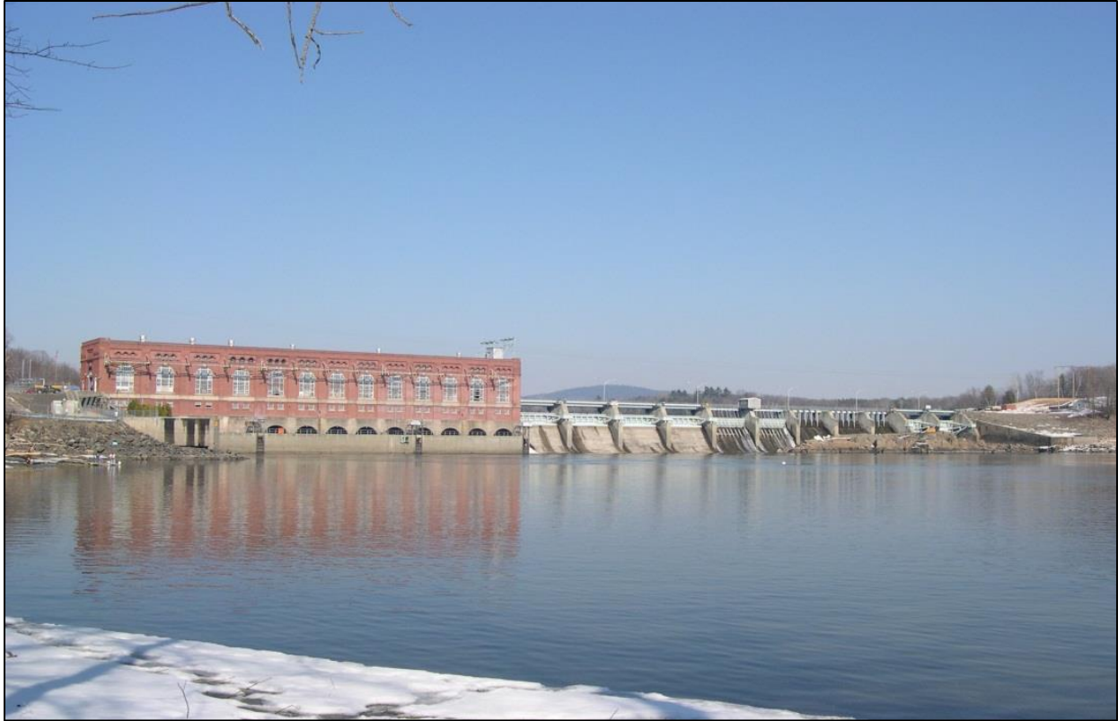
Figure 2.3-1 Powerhouse and dam looking upstream (fish ladder is not apparent).
