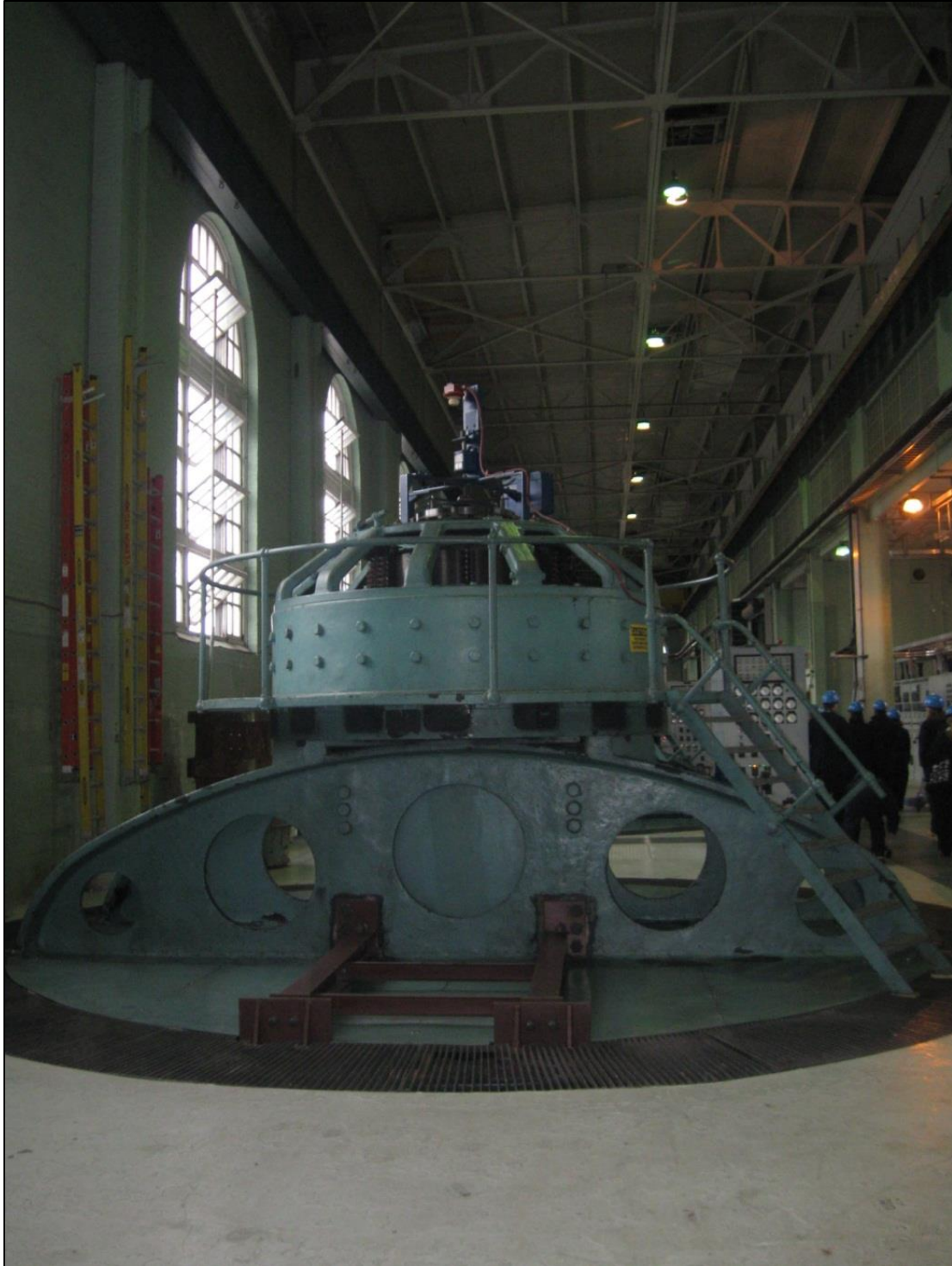
Figure 2.3-3. Generator Unit No. 10.
